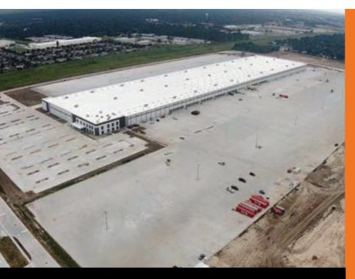
The largest OptiPave project at it's time of completion, a high performance OptiPave design reduces the amount of concrete needed.
