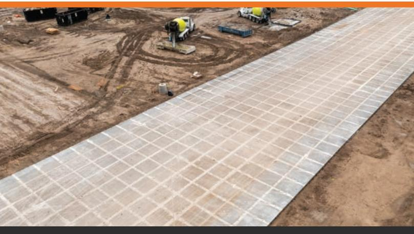
With a joint layout optimized by our OptiPave2 software, curling is reduced and axle loads are better distributed, reducing out-of-joint cracking.
